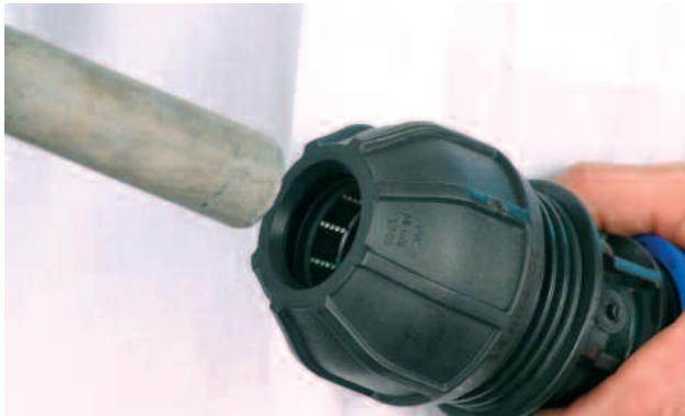
Introduce the pipe inside the fitting's body until it fully overtakes the universal D-Seal gasket and visually verify that the reference line, previously marked on the pipe, has effectively reached the prefixed position.
